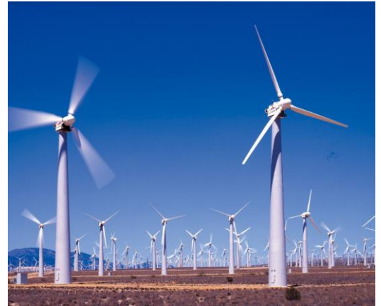
Wind Turbine Tower
