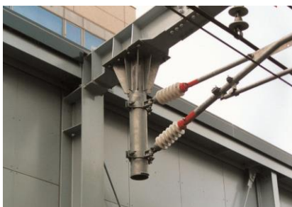
Steel Column Flange Stop
