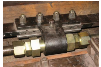
Switch Adjuster of Point
